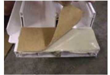
Correct placement of reinforcement.
